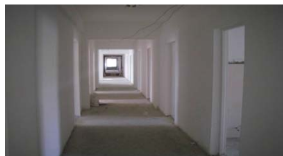
Works on the Reception Centre are almost complete
