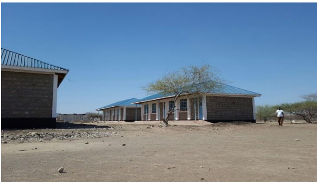
Photo: Completed construction of a pre-school in Kalobeyei
