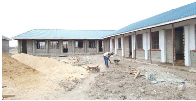
Photo: Ongoing construction of school B in Kalobeyei
