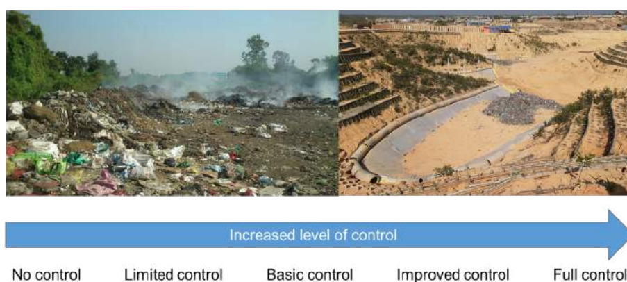
Figure 2: Illustration of two disposal sites along the level of control ladder. Left picture (ELS-EG, 2018) shows an open dumpsite without control. The right picture is the engineered sanitary landfill in Cox's Bazar (photo credit: UNDP) and shows an improved level of control with site planning, waste compaction and covering, and leachate management.
