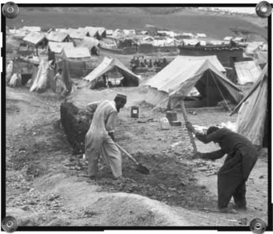
An estimated 170,000 Afghans have fled to Pakistan since September 2000, escaping both war and drought. The majority are housed at two large sites near the city of Peshawar, Shamshatoo and Jalozaï. Refugees prepare pit latrines at the New Shamshatoo camp. UNHCR/04.2001/C. Shirley
