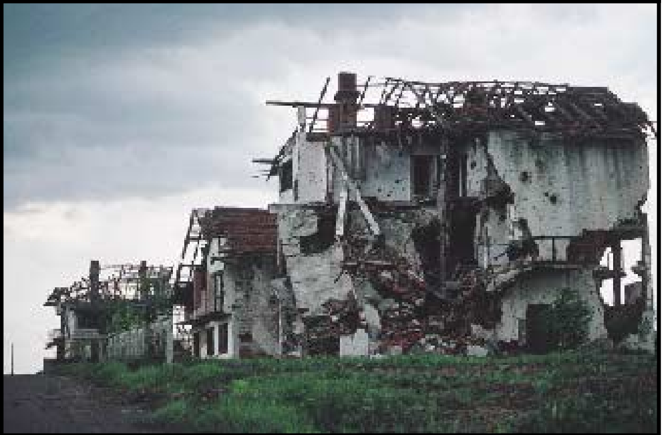
The price of war: Ruined houses in the Gradacac region of Bosnia, 1996.
