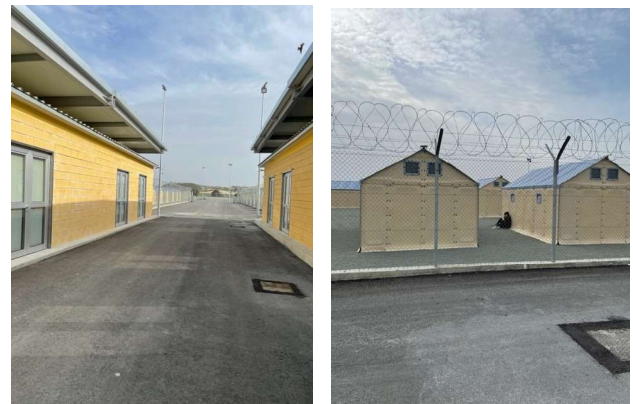
The Limnes centre before the onset of the refurbishment © UNHCR Cyprus
