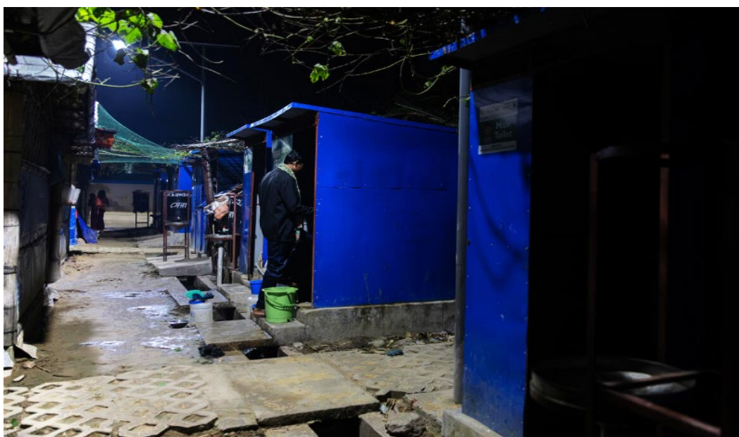
Improved waste management in Cox's Bazar contributes to more resilient WASH systems. © UNHCR/Shari Nijman
