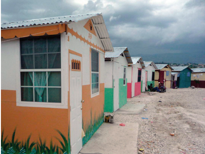
Transitional shelters built by Catholic Relief Services are expected to last between three to five years. Photo credit: Niek de Goeij, CRS.
