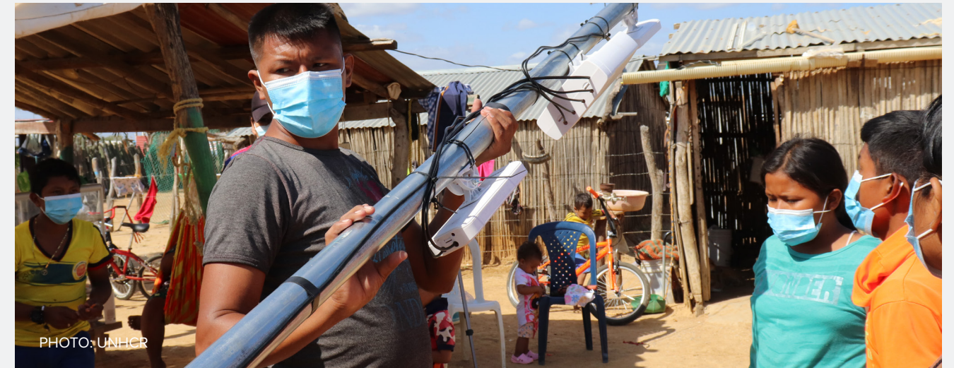
Internet infrastructure being set up for the community-led connectivity project – Colombia
