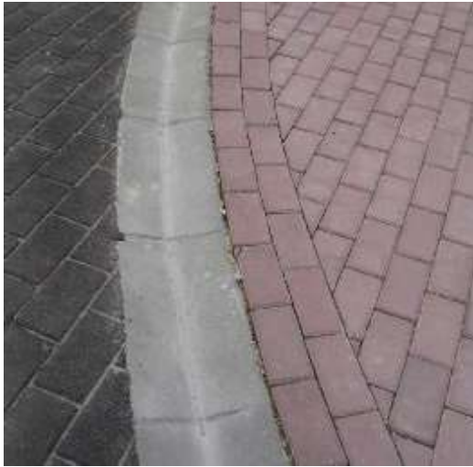
Sample concrete Drainage Channel
