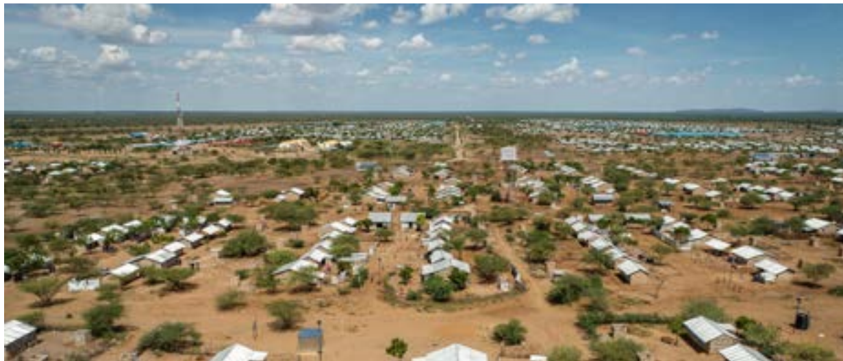
Kenya: aerial view of permanent houses constructed through UNHCR's CBI for Shelter Programme in Kalobeyei village.
