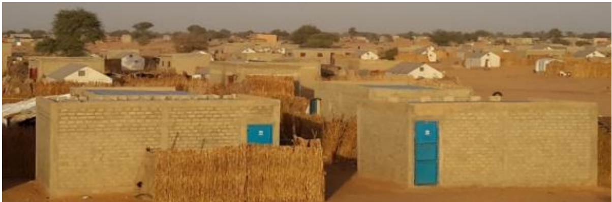
A view of homes built by UNHCR and partners, with hydraform (eco-friendly brick) material in Diffa. © UNHCR
