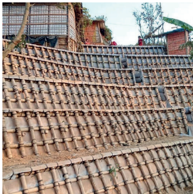
Murs-caisson en bambou. Inter-Sector Coordination Group, 2022
