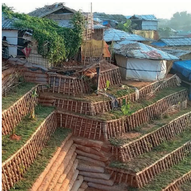
Murs-caisson en bambou. Inter-Sector Coordination Group, 2022
