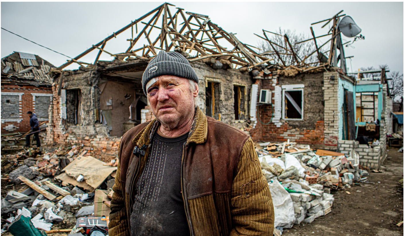
Artem stands near his damaged home in Kramatorsk, eastern Ukraine, where daily shelling has become the norm. After a recent attack destroyed much of his house, UNHCR and partner Angels of Salvation helped repair part of the roof through the 'Workshop on Wheels' initiative. "I was of course affected, but there is nothing you can do about it. Life now goes this way," he says. © Angels of Salvation/Oleksiy Gutnyk
