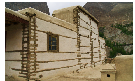
Traditional Bhattar Construction, Pakistan, Foto © T. Schacher
