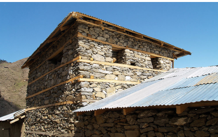
New Bhatar (Stone, Timber) Construction, Pakistan, (Foto © T. Schacher)
