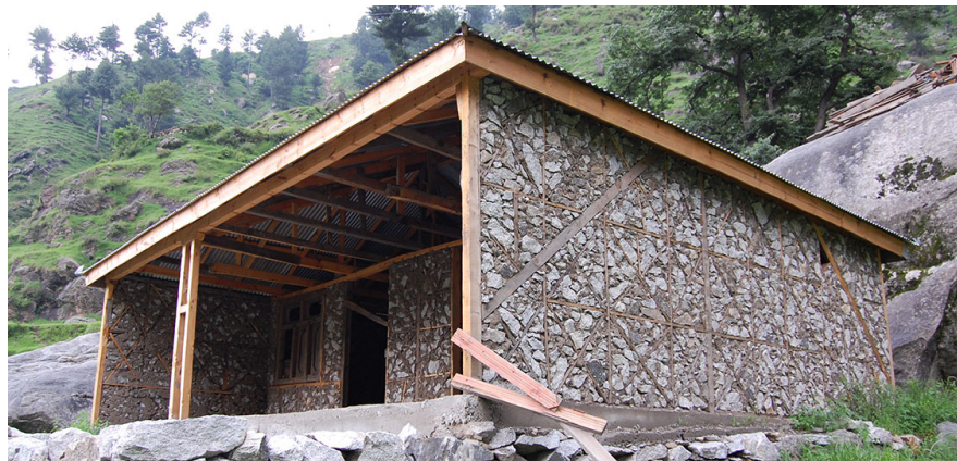
New Dhajji (Stone, Timber) Construction, Pakistan, (Foto © T. Schacher)
