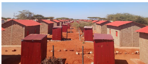
33 housing units constructed in 2025, in Bokh Refugee Site, Ethiopia. © UNHCR
