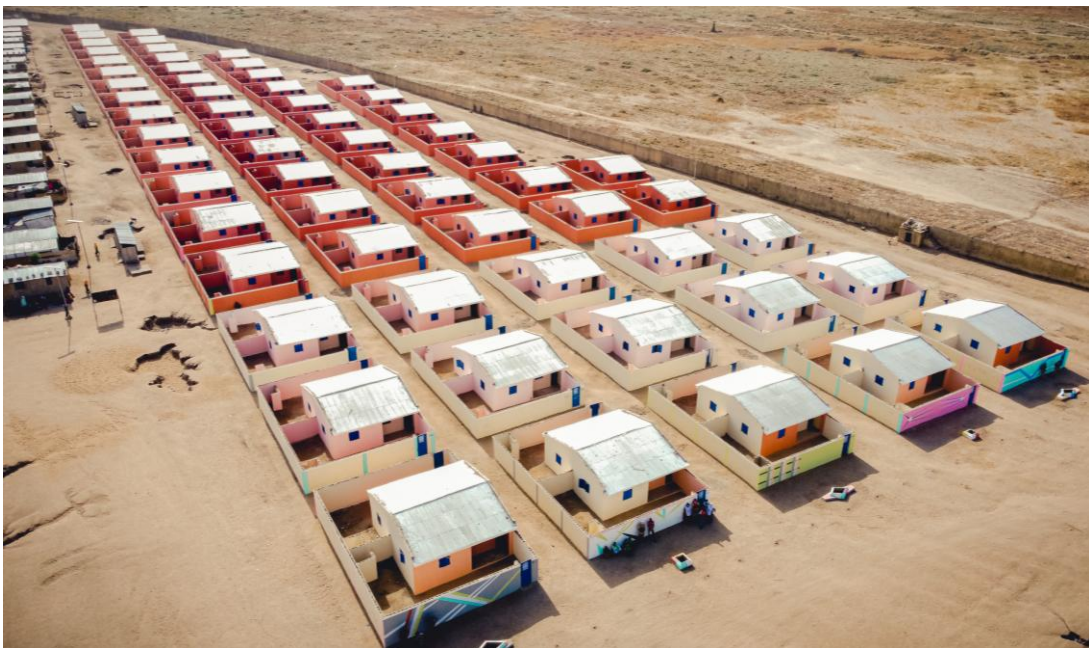
In Nigeria, UNHCR, in partnership with the State Government through the Ministry of Rehabilitation, Reconstruction, and Resettlement, delivered 450 housing units to refugee returnees and vulnerable Nigerian populations
