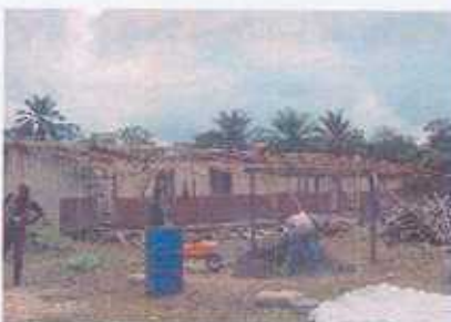
Renovation of the Sekonodu Public School, Lofa
