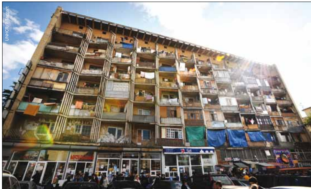
IDP collective centre in former hospital building, Tbilisi, Georgia. An estimated 148 families live in this hospital complex which suffers from widespread rat and insect infestation and falling masonry.
