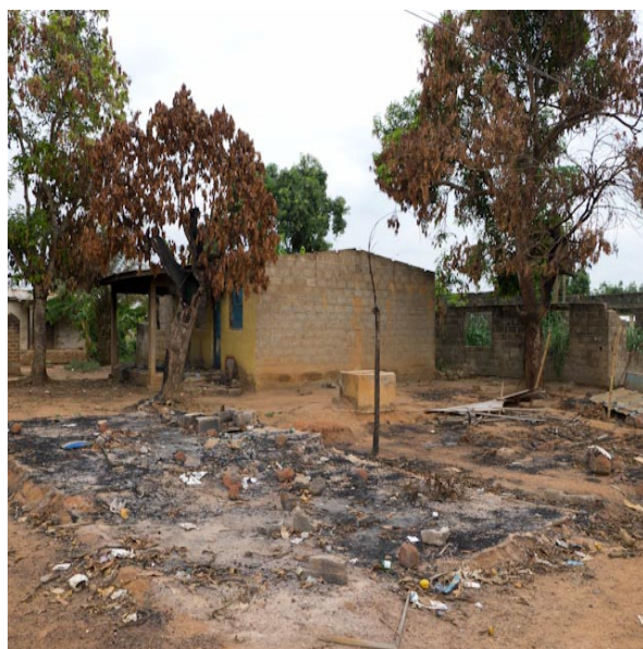
Destroyed houses in Quartier Carrefour, Duékoué, Côte d'Ivoire. (UNHCR/Dewoelmont /2011)
