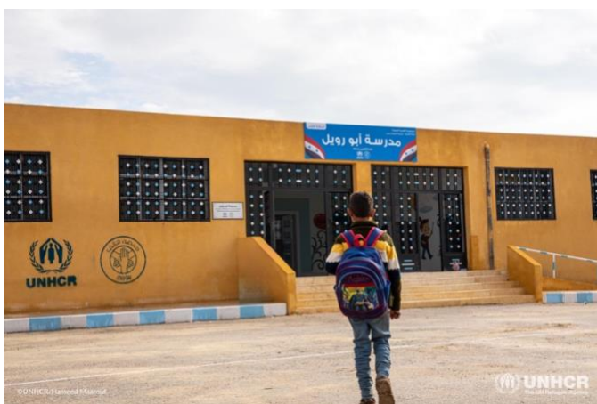
Abu Rweil Elementary School affected by the February 2023 earthquakes was repaired by UNHCR and is ready to welcome students again. ©UNHCR/ H.Maarouf
