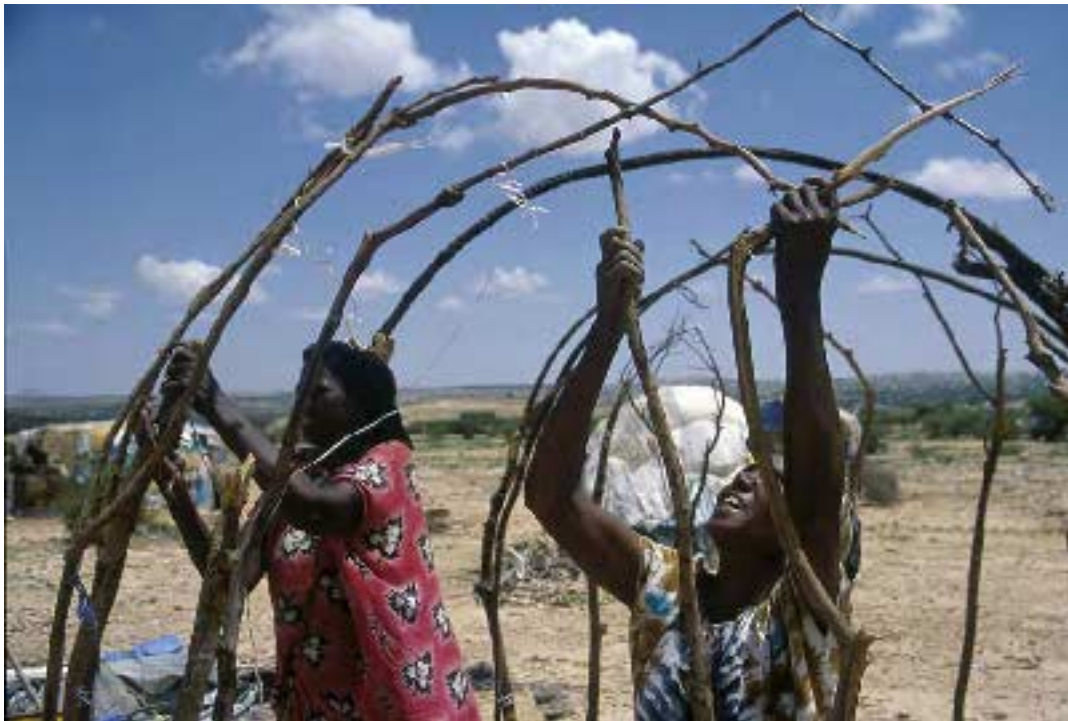
Somalia/IDP women constructing shelters/Kondahar IDP Camp, UNHCR/L.Taylor
