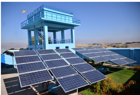
Afghanistan. UNHCR installs solar-powered community water network. ©UNHCR/Mohammad Anwar Danishyar
