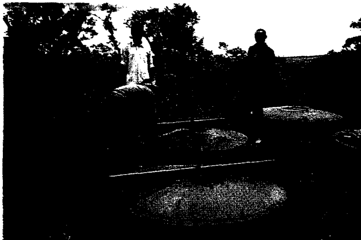
Plate 16 - Construction of a cement dome slab for a latrine at Musuhura camp (Tanzania, Ngara).
