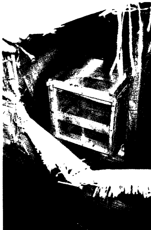
Plate 12 - Fly traps installed on the defecation hole of a latrine.
