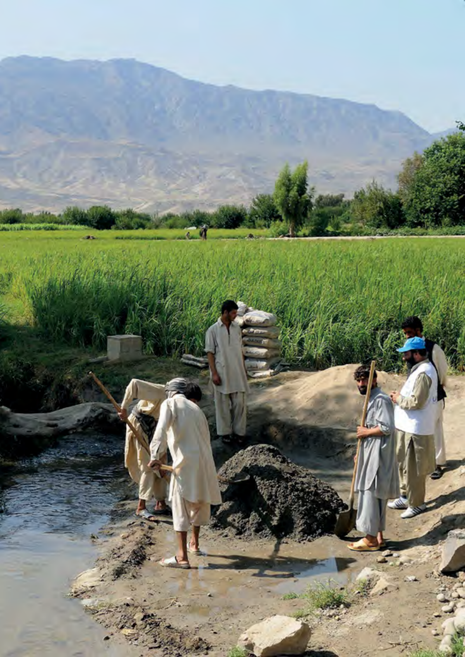
◀ Afghanistan / A joint UNHCR-WFP irrigation project in Farmankhel provides returnees with arable land for growing staples and cash crops. UNHCR / R.Arnold / 2008
