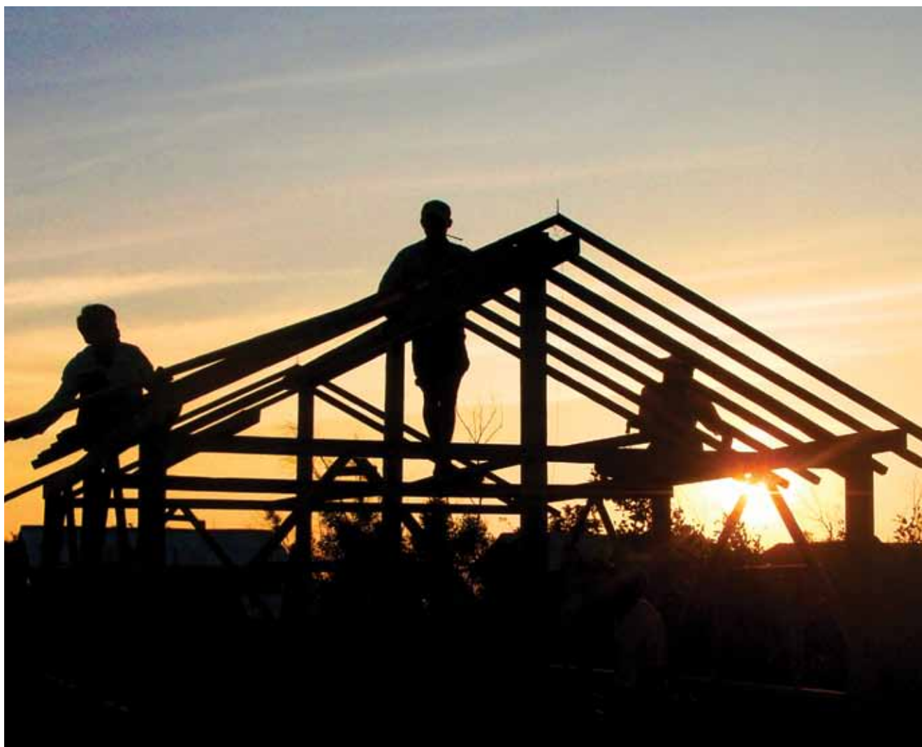
MYANMAR: Cyclone Nargis hit Myanmar in May 2008, killing 140,000 and displacing 800,000. The Norwegian Refugee Council is rebuilding homes in the hardest hit area. Diagonal beams fitted to the house frame are among the new building techniques applied, in order to make the new homes resistant to future cyclones. (Photo: Martin Suvatne/NRC)
